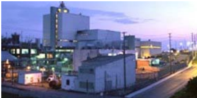
Figure B1– 4 Port Hope conversion facility.
