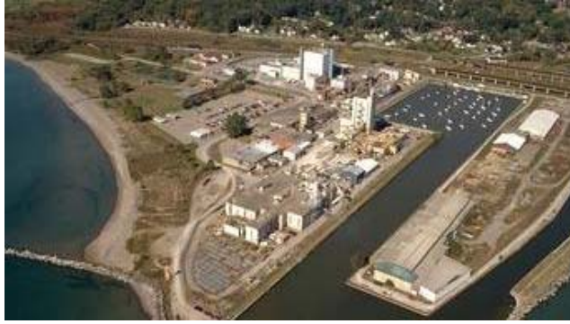
Figure B1– 3 Port Hope Conversion and Fuel Fabrication Plant (Cameco) in Ontario, Canada.
