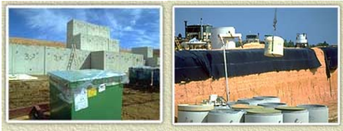
Figure G3-5. Waste placement in landfill at Chem-Nuclear Systems Barnwell (South Carolina) site (Chem-Nuclear Systems, LLC 1997).
