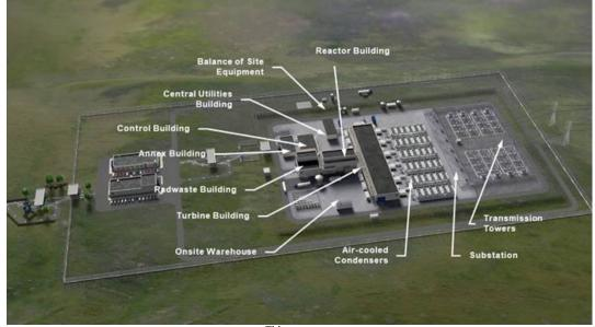
Figure A-7 Conceptual site layout of VOYGR<sup>TM</sup> (Courtesy of NuScale Power)
