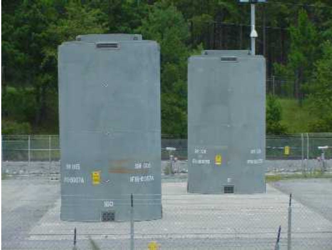
Figure G-4. Holtec International HI-STORM Dry Storage Casks on storage pad (Note vertical storage). Figure copied from Holtec International Web site.
