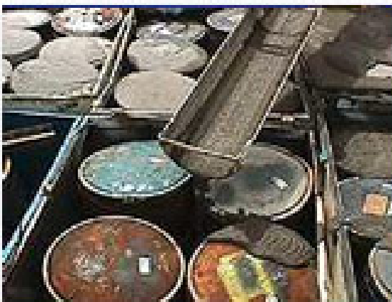
Figure G-8. Filling voids around drums at Envirocare Facility in Utah. Figure copied from Envirocare Web site.
