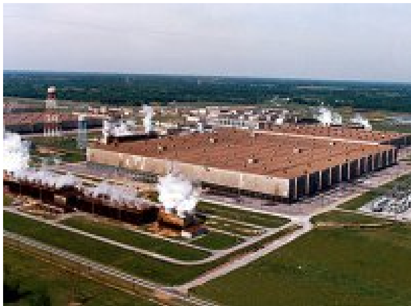
Figure C1-7. United States Enrichment Corporation Gaseous Diffusion Production Building.
