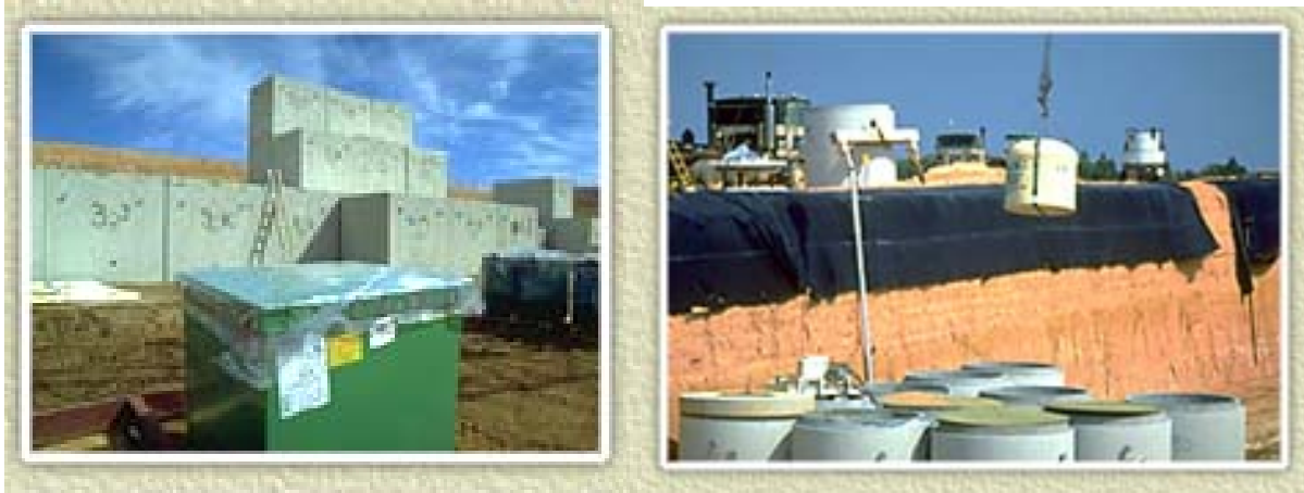
Figure G-11. Waste placement in landfill at Chem-Nuclear Systems Barnwell site. Figure copied from Chem-Nuclear Systems Web site.
