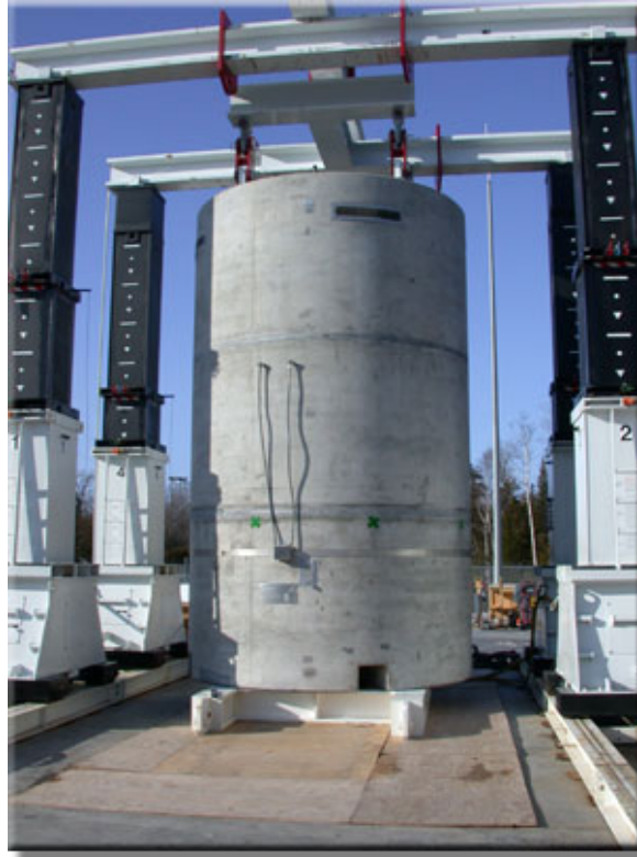
Figure G-6. BNG Fuel Solutions vertical cask lift. Figure copied from BNG Web site.
