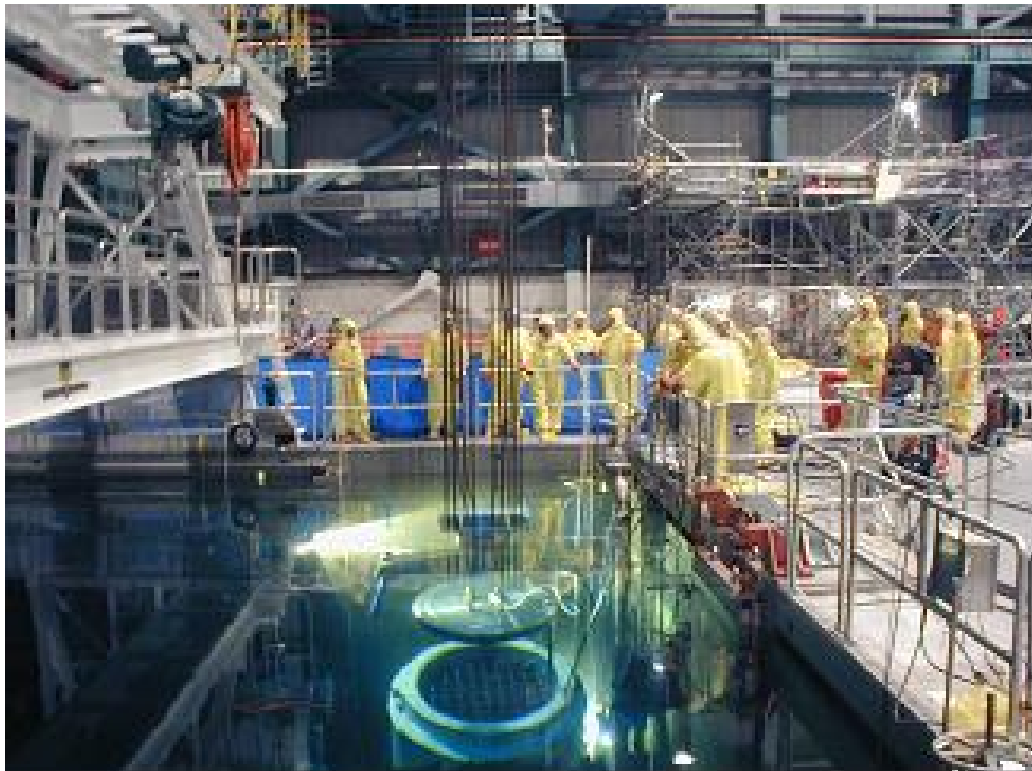
Figure E2-5. Cask for dry fuel storage being closed under water for shielding protection.
