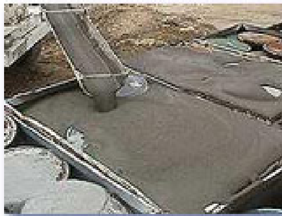
Figure G-8. Filling voids around drums at Envirocare Facility in Utah. Figure copied from Envirocare Web site.
