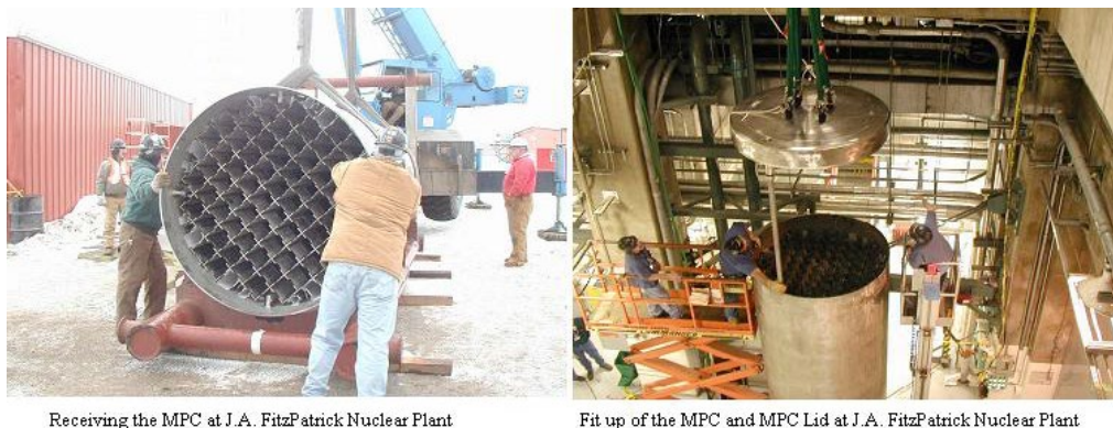
Figure G2-1. Holtec International fuel storage canister to be loaded with fuel assemblies. Figure taken from Holtec International Web site.
