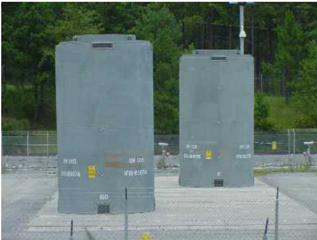
Figure G2-3. Holtec International HI-STORM Dry Storage Casks on storage pad (note vertical storage). Figure taken from Holtec International Web site.
