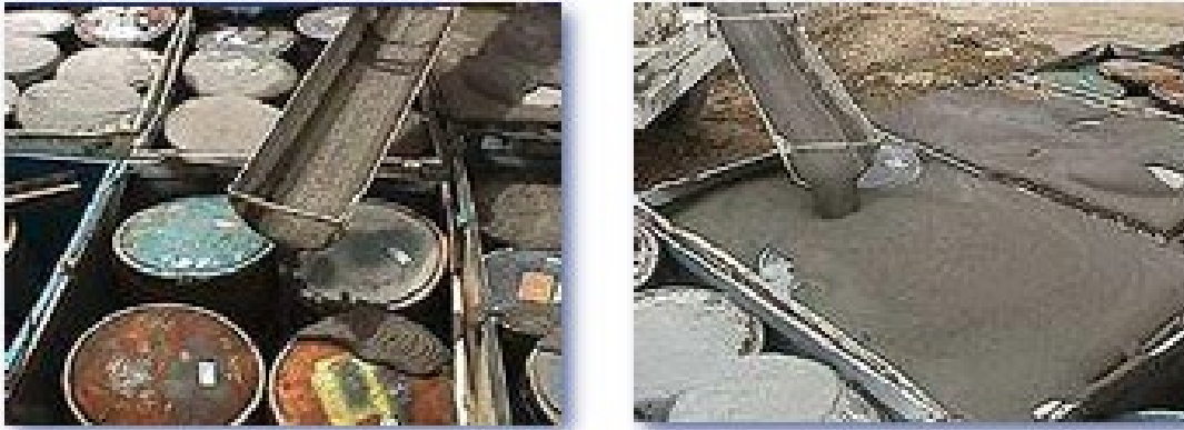
Figure G3-2. Filling voids around drums at EnergySolutions Facility in Utah. Figure taken from EnergySolutions Web site.
