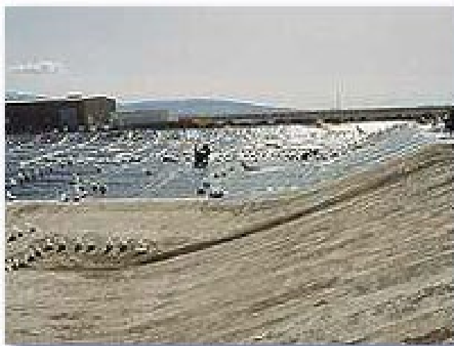
Figure G3-4. Landfill disposal cell at EnergySolutions (Note line and leachate collection piping). Figure taken from EnergySolutions Web site.
