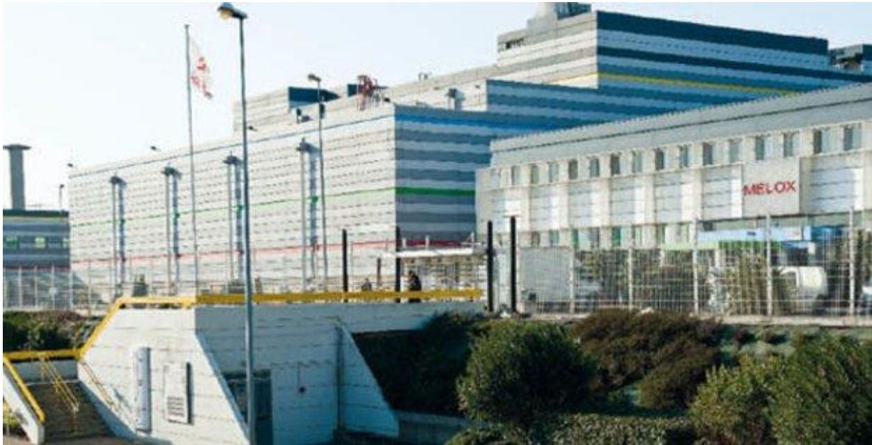
Figure D1-2.2. MELOX LWR-MOX Fuel Fabrication Facility in France (ORANO 2021).
